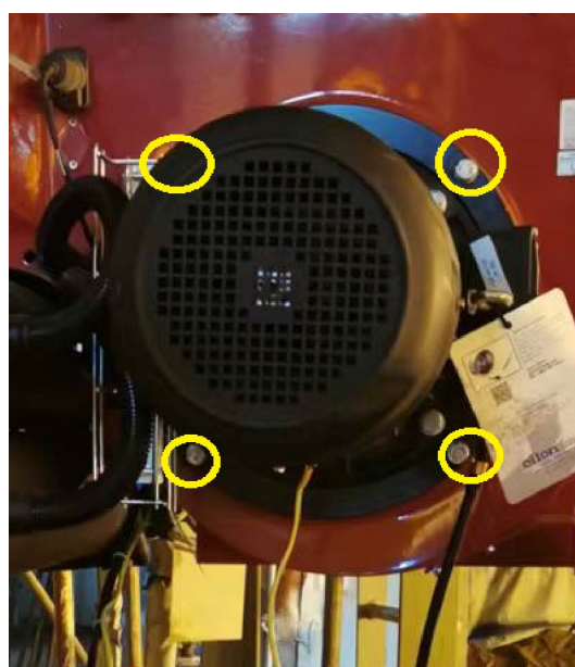
Fastening screws, fan motor assembly 3 ver. 1
